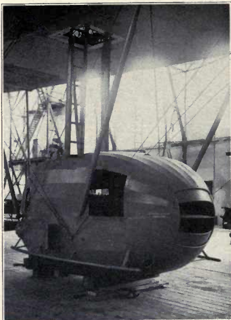
The "DELAG" Passenger Zeppelin "Bodensee." Front and rear views of rear power gondola. Note radiator temperature control and ladder.
